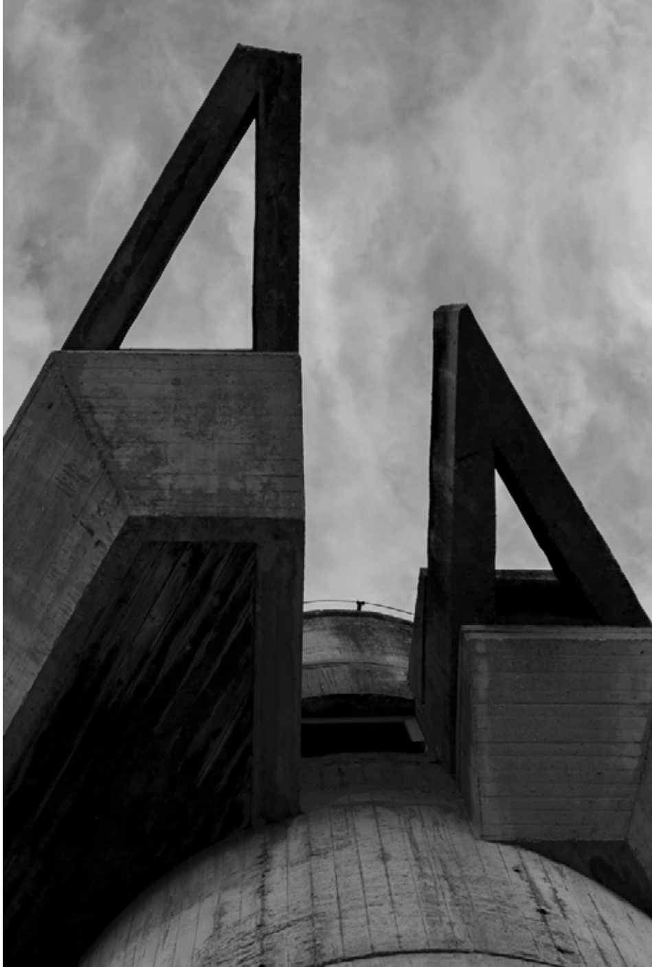
Hydrometeorological Service Building, photo credit Mattia Pandolfo
